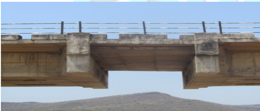
Photo no. 5 - Deflected suspended span on left side
