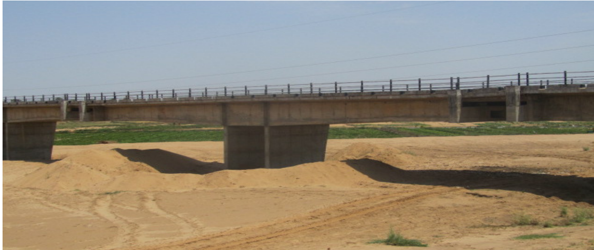
Photo no. 1 - settled pier P10
