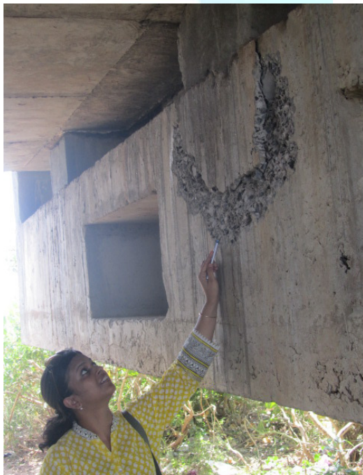
Photo no. 2 - Tip of cantilever span
