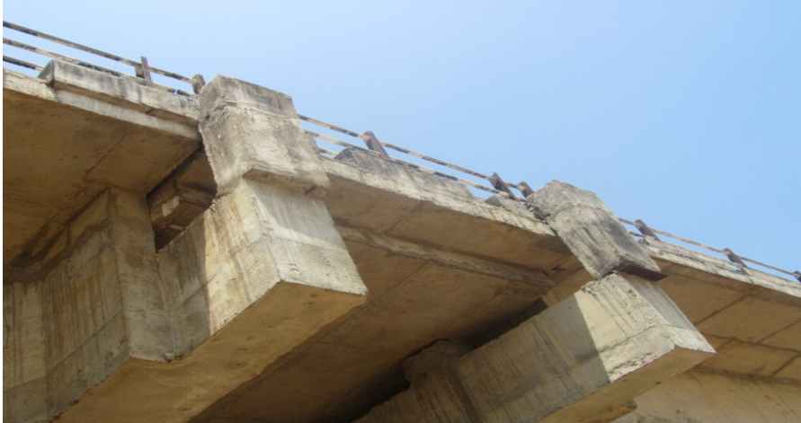
Photo no. 3 – Protection of suspended span
