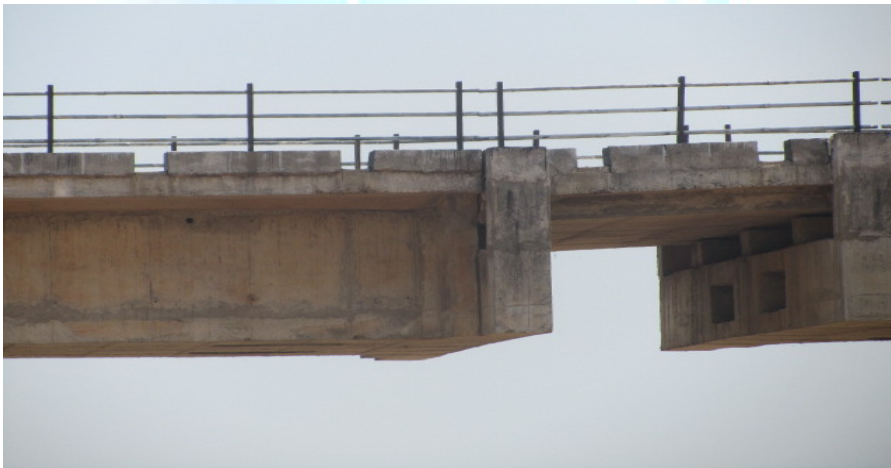
Photo no. 4 - Deflected suspended span on right side
